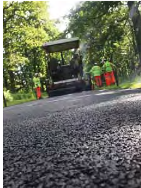
Maintenance work, image courtesy of Asphalt Industry Alliance
