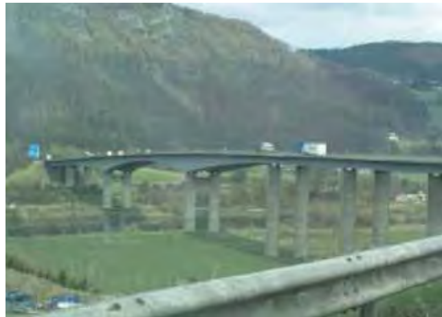
Critical infrastructure, image courtesy of Atkins
